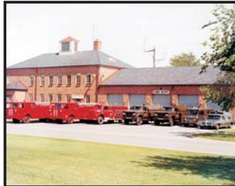
Letterkenny fire department is located close to the main gate and next to the administration building.
